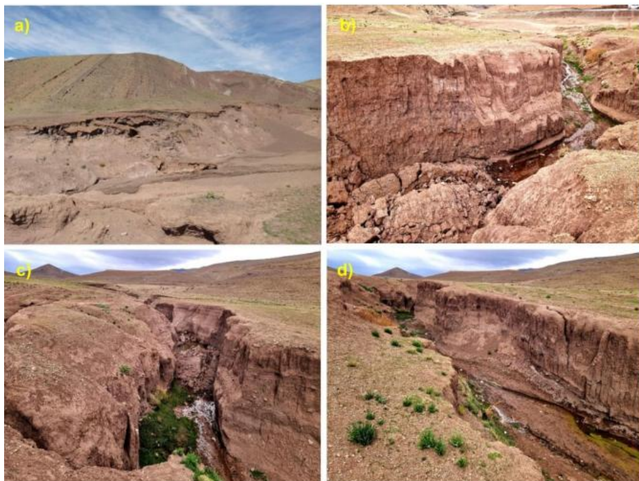
Figure 12. (a) Bank undercutting and slope failures in the upstream part of the Ouirghane sub-basin (Taghighacht sector). (b), (c), and (d) Deep gully incision and vertical bank retreat in the Tingagou area (Lakes Plateau), illustrating progressive channel deepening and lateral erosion
